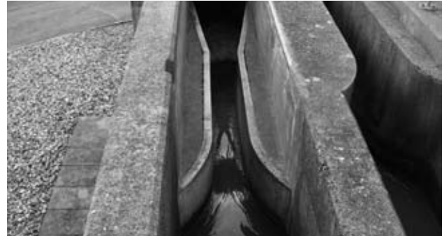
Venturi flume: Typical 3/2 power law
